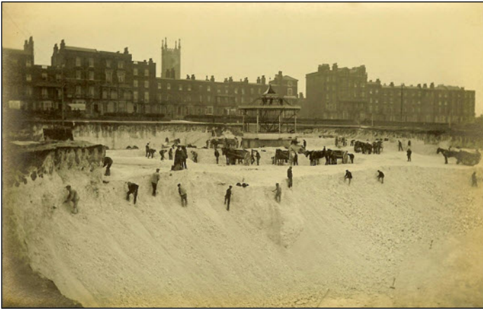
Work commences in removing the huge quantities tons of chalk from the site which were dug out by pick and shovel - no mechanical diggers were available in those days. The chalk material was used as infill for the building of the adjacent promenade. Note the continued presence of the bandstand in the above pictures. Perhaps it was originally intended to retain the bandstand in its original position?
