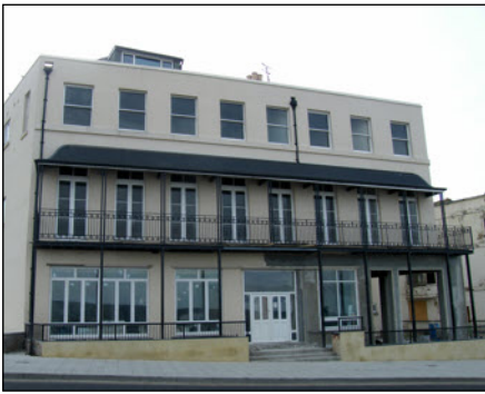
The Arcadian, Fort Hill (Refurbishment)
