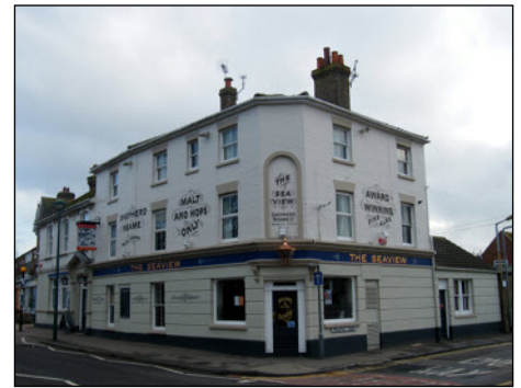
The Seaview Hotel, Station Road Birchington (Refurbishment)
