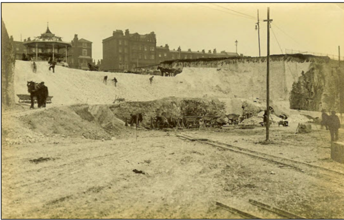
Work commences in removing the huge quantities tons of chalk from the site which were dug out by pick and shovel - no mechanical diggers were available in those days. The chalk material was used as infill for the building of the adjacent promenade. Note the continued presence of the bandstand in the above pictures. Perhaps it was originally intended to retain the bandstand in its original position?
