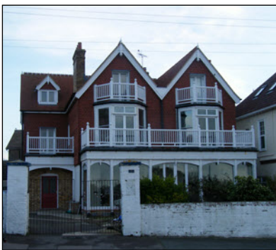
71 Sea Road Westgate-on-Sea (Replacement of balconies, etc)
