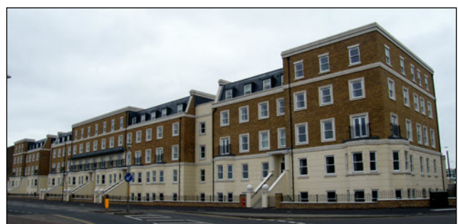
Burlington Place, Eastern Esplanade, Cliftonville (New development)
