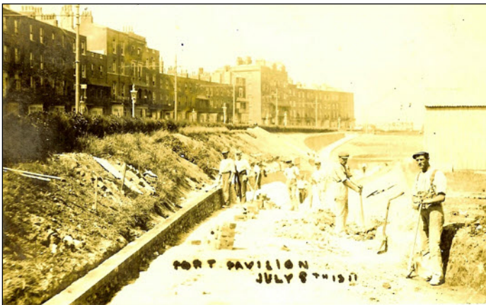
The carriageways begin to take shape - 8th July 1911
