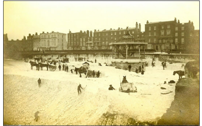
Work commences in removing the huge quantities tons of chalk from the site which were dug out by pick and shovel - no mechanical diggers were available in those days. The chalk material was used as infill for the building of the adjacent promenade. Note the continued presence of the bandstand in the above pictures. Perhaps it was originally intended to retain the bandstand in its original position?
