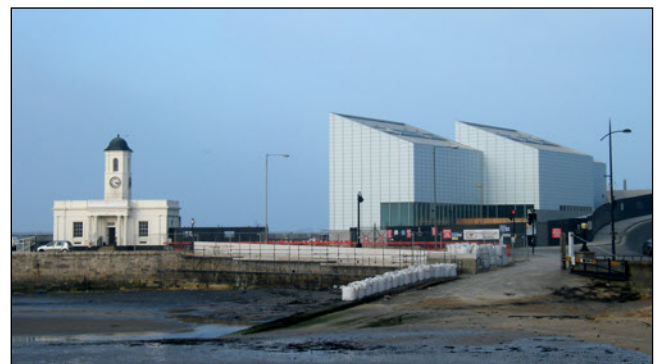
Turner Contemporary (Construction of new art-gallery)
