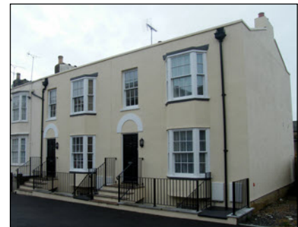
5 & 6 Caroline Square, Cliftonville (Refurbishment)
